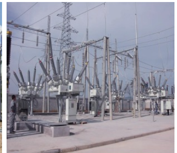
Single busbar arrangement
